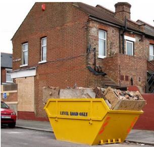
How do the calculations deal with removal at the end-of-life? Construction practices vary widely and some products are harder to recycle due to their material or multi-layer construction. With the exception of the brass fittings included in the typical configuration, the EPDs assume the building contractor would skip and send the waste to landfill or incineration.
