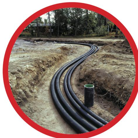
Choice of bedding and backfill materials, design of cover depth to accommodate traffic loadings and compaction requirements all follow the same principles as polymer pipes for water supply systems. Manufacturers provide detailed guidance on this aspect.
