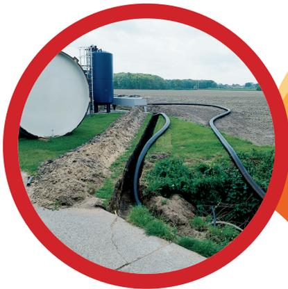
**Open trench** – this is the most common technique. Narrow trenching can be used if the installer can work safely to make any joints. Damage to the jacket pipe from poor handling can be repaired using a suitable repair set available from the manufacturer.
