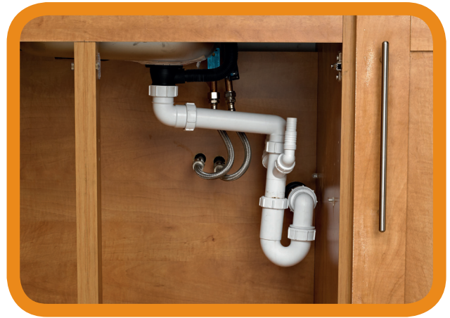
Domestic sink with water-seal trap
