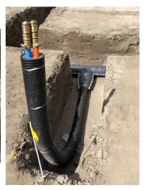
Choice of bedding and backfill materials, design of cover depth to accommodate traffic loadings and compaction requirements all follow the same principles as polymer pipes for water supply systems. Manufacturers provide detailed guidance on this aspect.
